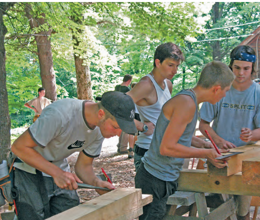
At left, French apprentices directed by Heartwood School student Ben Theriault (at right in bandanna) lay out rafters in Washington, Mass. At top, Martin Lorentz, seated at the Millers Falls boring machine, and Boris Noël, standing at right, compagnons who came from Troyes to help supervise the 20 French apprentices (or rabbits). Above, apprentices intently shaving pegs split out from block.
