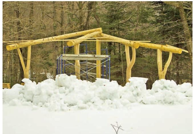
1 At top, reciprocal-framed gazebo 32 ft. in diameter, winter-built of Eastern white pine logs in northern New England, purlins in place before roofing over. Forked posts provide transverse bracing, low walls shear bracing in alternate panels. Not part of original design, two-tiered stainless steel cupola 8 ft. 6 in. dia. covers aperture and will be supported by temporary posts during winter months to resist added snow load.
