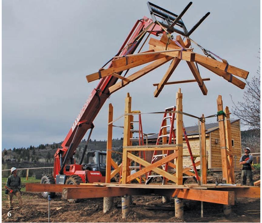
5 First and seventh rafters spread to allow insertion of eighth, Jake Amadon considering next move. Repositioning and application of appropriate force won the day.
