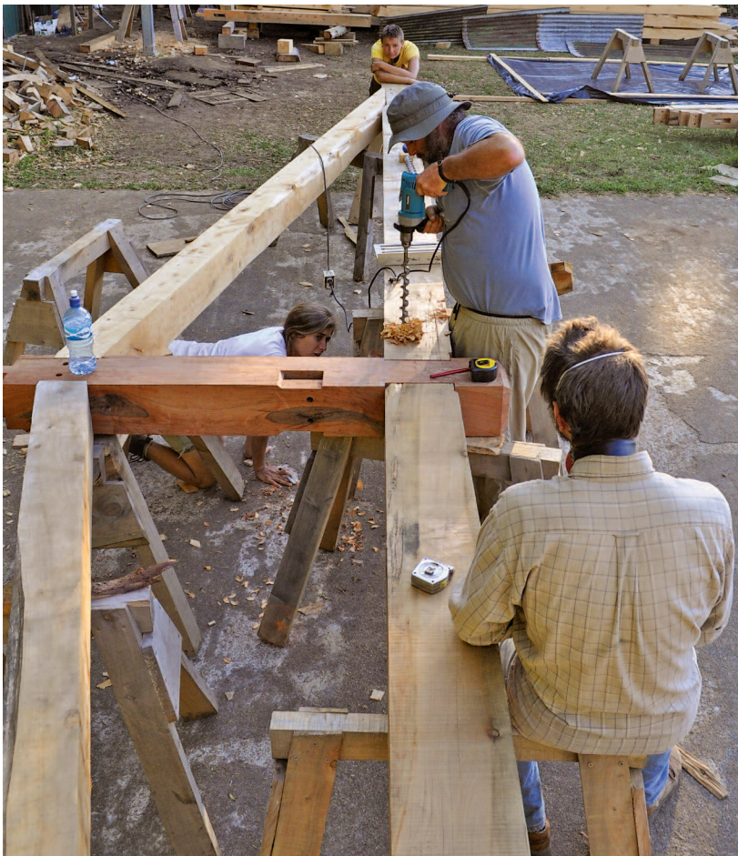
At top, raising complete at courtyard end of frame. Above left, truss assembly on horses: David Hooke drills for spline pins while assistant eyeballs plumb and author checks for drillbit blowout. Above right, swervy brace accommodates procedural error in great style.
